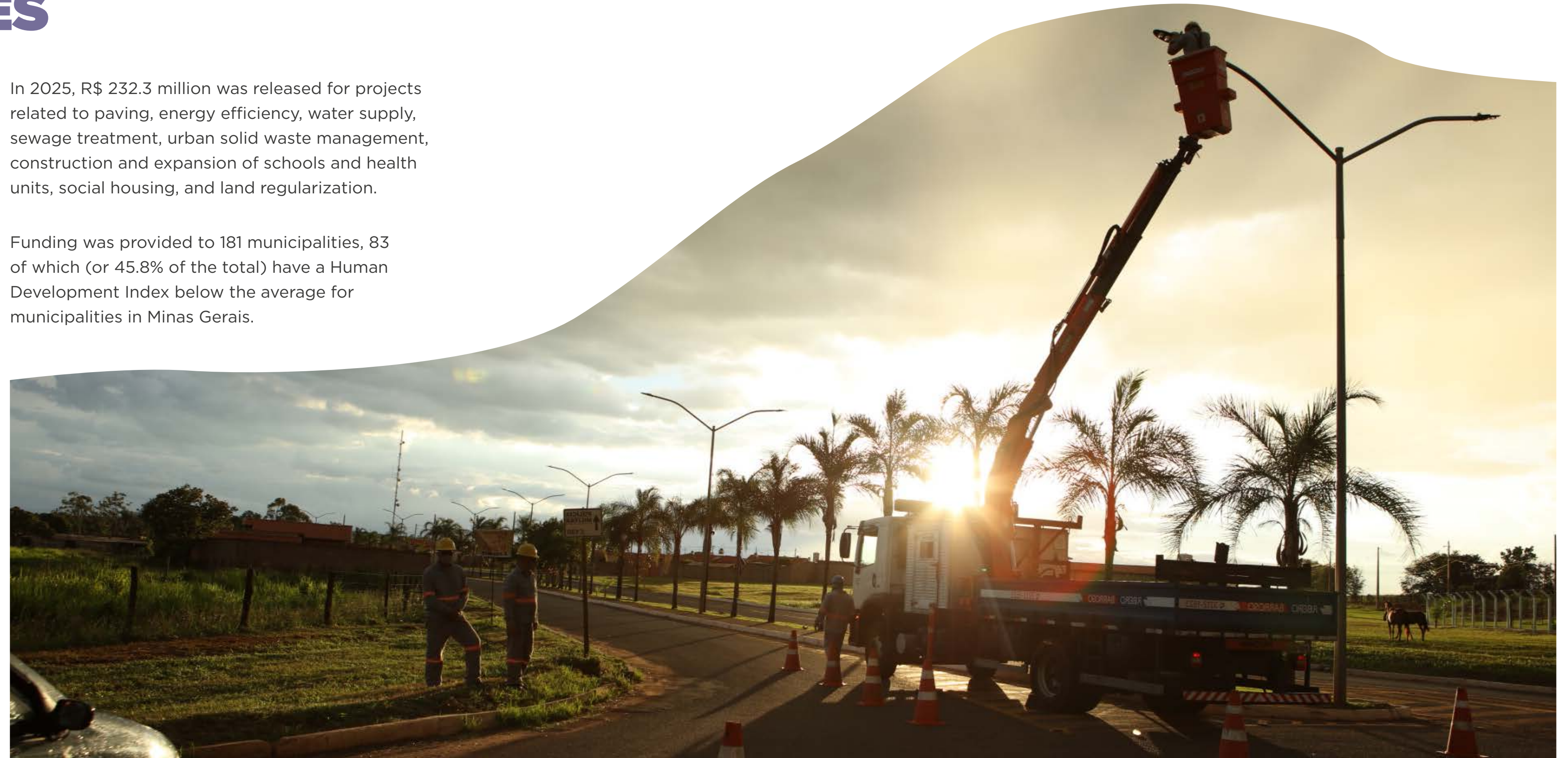
Public lighting project
